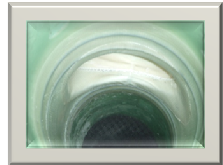
Figure 3: Structural Main/Lateral CIPP
